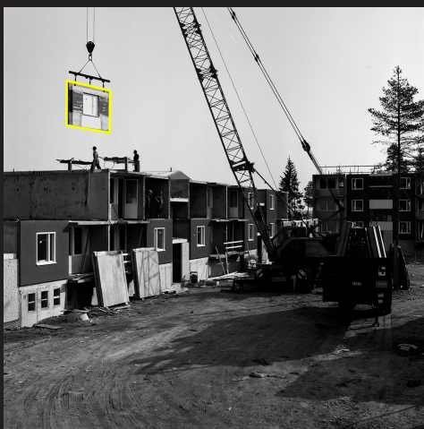
Top: Sune Sundahl Installation of large concrete panels in residential buildings, 1967–1968 ArkDes photo collection
