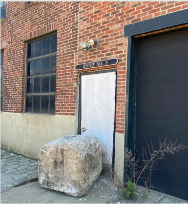
Doors blocked from trespassers
