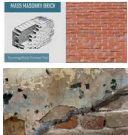
**This page, top right: Typical Mass Masonry Brick Construction.** Source: International Union of Bricklayers and Allied Craftsmen
