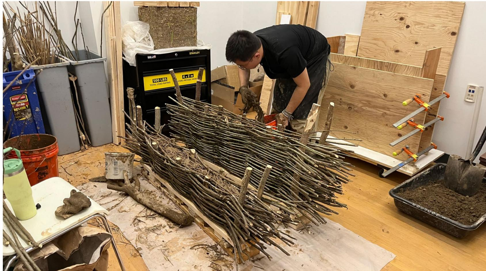
After the building process, the Streamco willow whips start to take root and germinate, which proves the possibility of the straw clay in wattle frames to be a living and evolving system.
